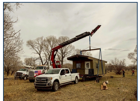
Delivered & placed on site
